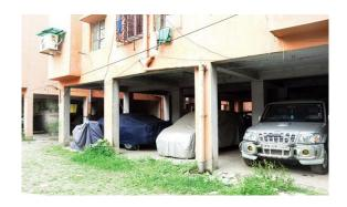
Figure no-1 Open Ground Storey (courtesy -www.telegraphicindia.com)
