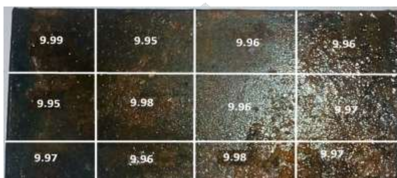
Fig 4.1: Thickness marking on corrode plate after measurement of specimen A
