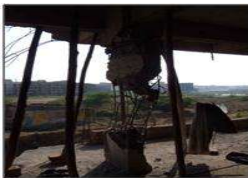
Fig.5 Micro concreting
