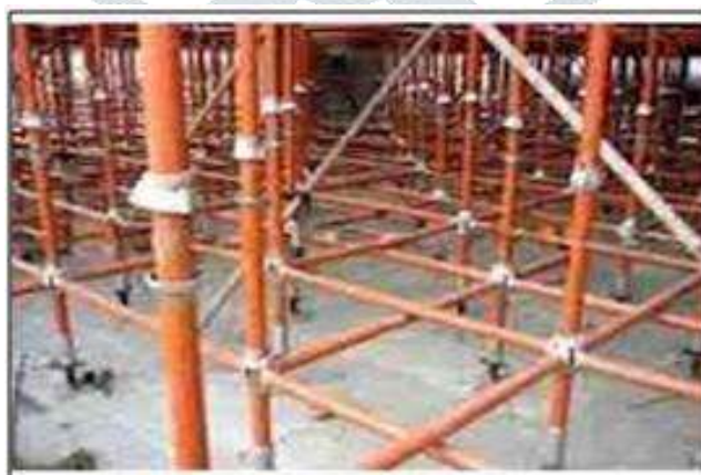
Fig.4 Erection of scaffolding
