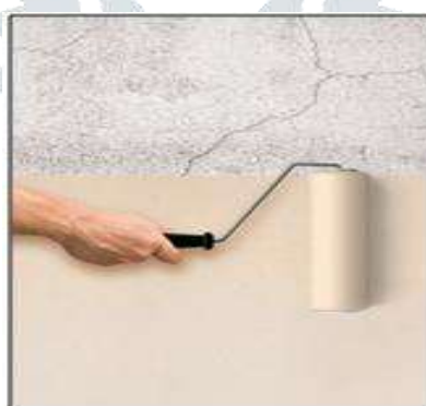
Fig.7 Crack Bridging coating
