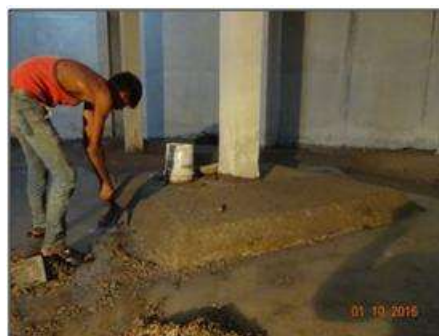
Fig.8 Water proofing work inside the ESR
