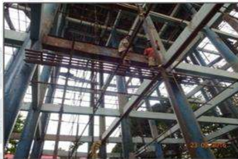
Fig.6 Erection of scaffolding
