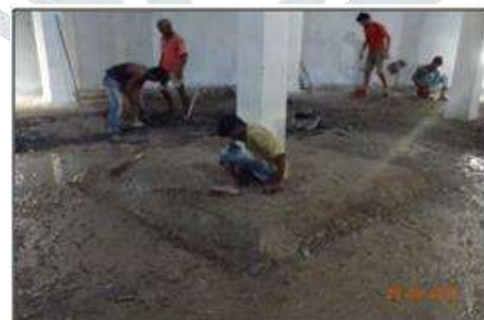
Fig.7 Repair work inside the ESR
