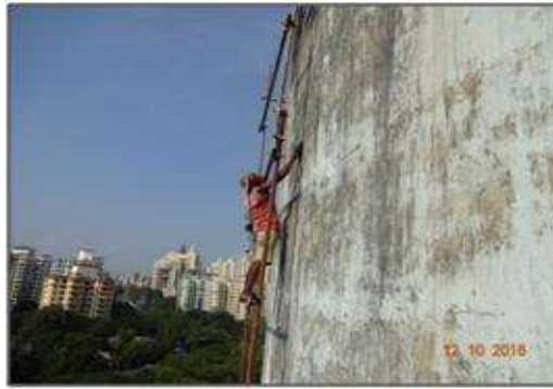
Fig.9 External repair work
