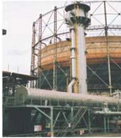
Fig.1 Kalina Cycle Installation
