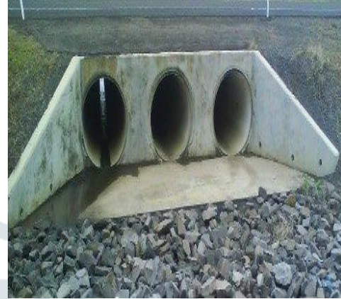
Figure 0-1 Box culvert Figure 2 Pipe culvert
