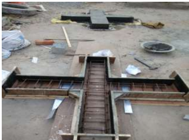
Fig 8 Casting Of Joints
