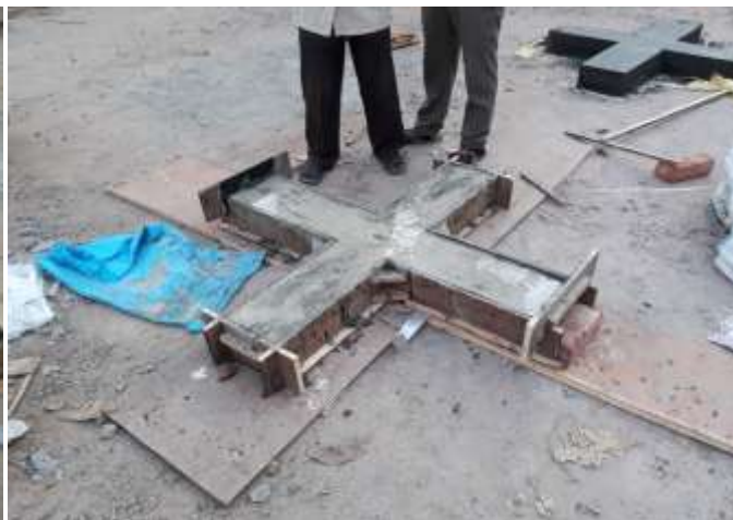
Fig 9 Curing Of Beam Column Joints
