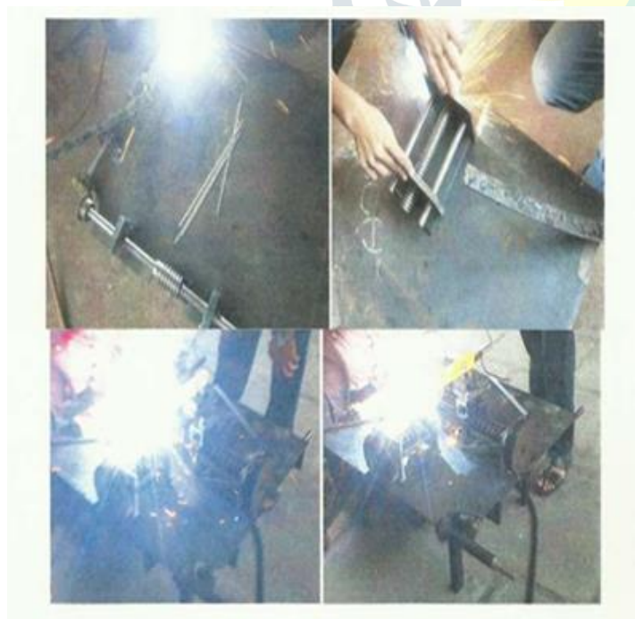
Figure 5: Welding of Components
