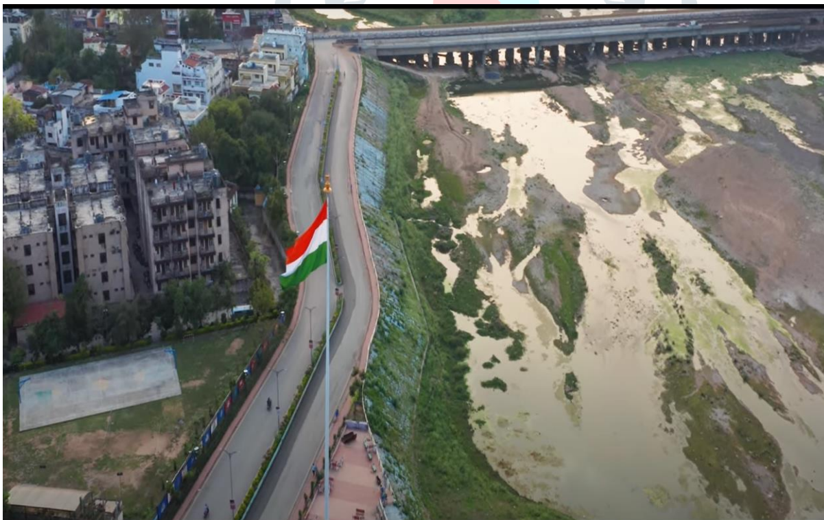
Fig.5 Drone Photography for Indra Bridge to Lingyadh Bridge
