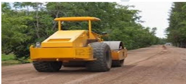
Photograp : Surface compaction
