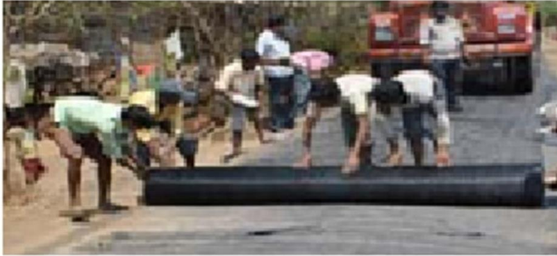
Photograph. - Fabric Unrolled and Overlapped (or seamed)
