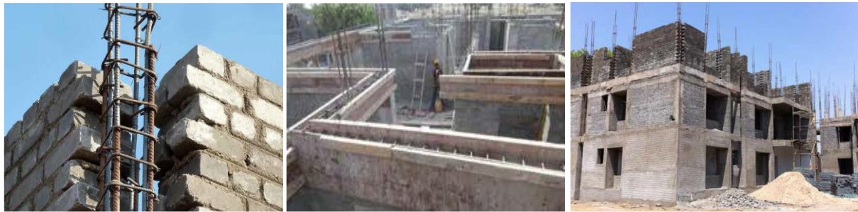
Fig No.6 Constructions of Confined Masonry Buildings (Ref. Campus on Sabarmati 18 )
