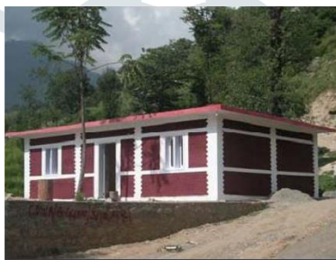
Fig. No. 1 Finished confined masonry structure (Ref. Zulqarnain A. S. et. al 2 )
