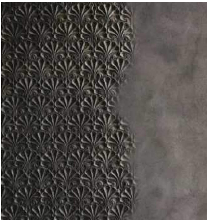
Figure 12: Using blocks while plastering
