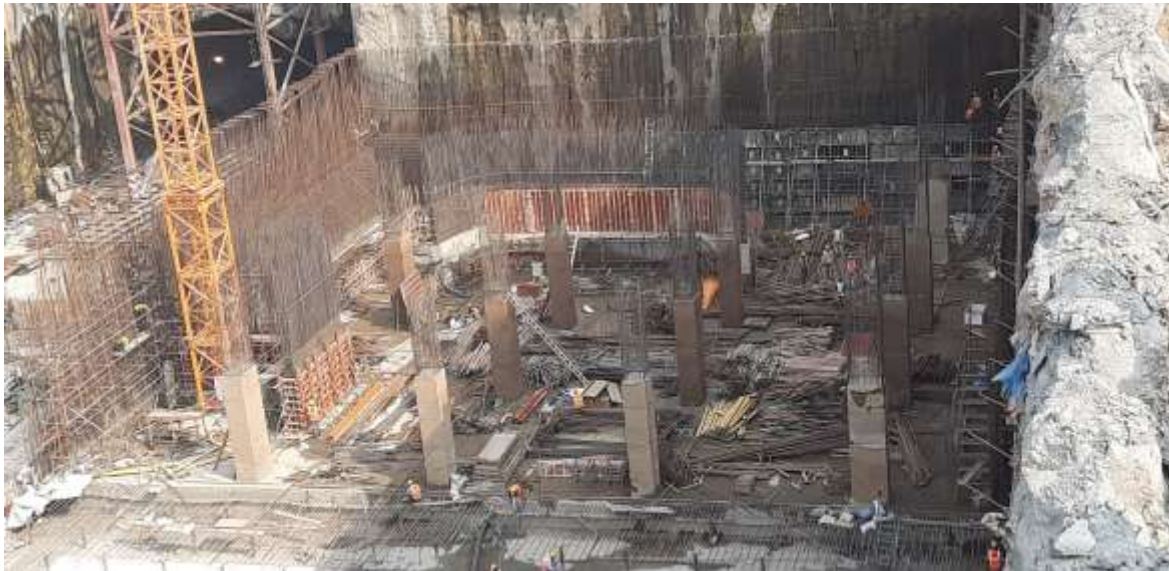
(Photo No.02: Scaffolding on site)
