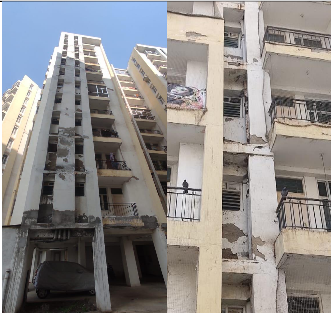
Fig: -1 Visual inspection of the building.
