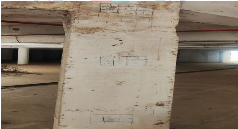
Fig: -9 Rebound Hammer Testing on Column
