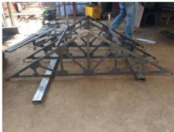
Fig 5.3 Assembling the purlins
