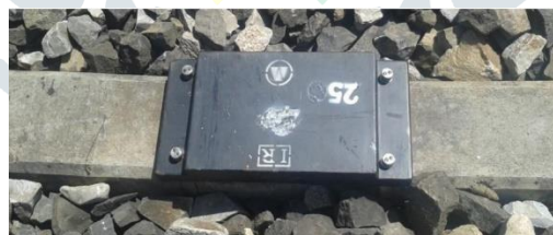
Figure 5: RFID tag fixed on a sleeper
