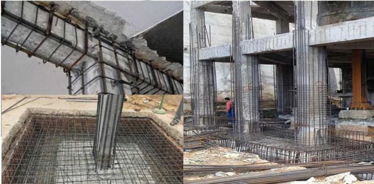
Fig.6 retrofitting of columns building
