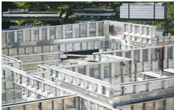
Fig 2.4 Aluminium Formwork during construction
