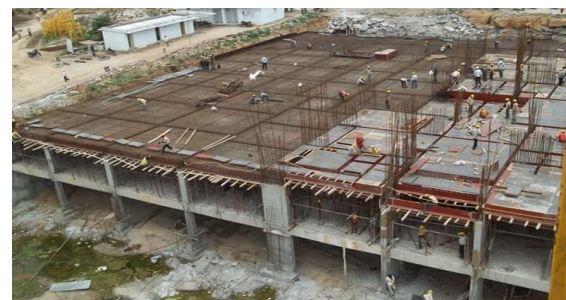
Fig 2.2 Aluminium Formwork during construction
