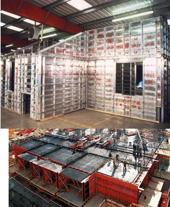
Fig 2.3 Aluminium Formwork during construction
