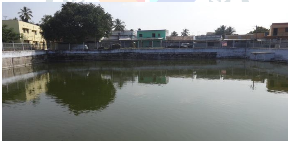
Figure 2.1: Current view of the Temple tank-I, Karamadai Temple tank, Coimbatore
