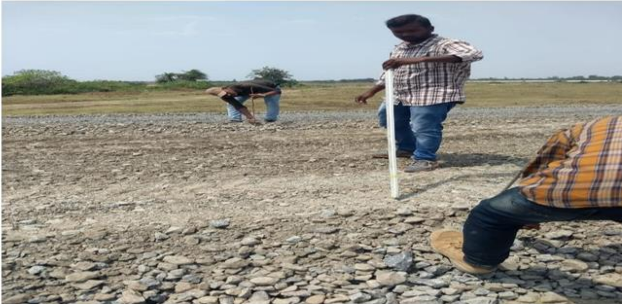
Fig 2: Leveling on road
