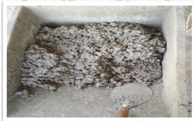
Fig No. 1 Concrete mix
