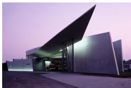
Figure 2- Vitra Fire Station, Weil am Heim, Germany
