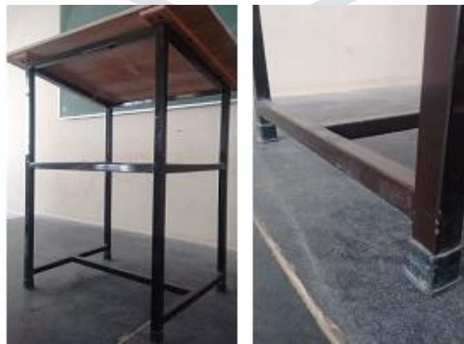
Fig. 2. Damaged Bush
