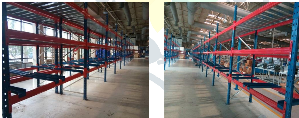
Figure 4: Photograph of U-power layout (work in progress picture)
