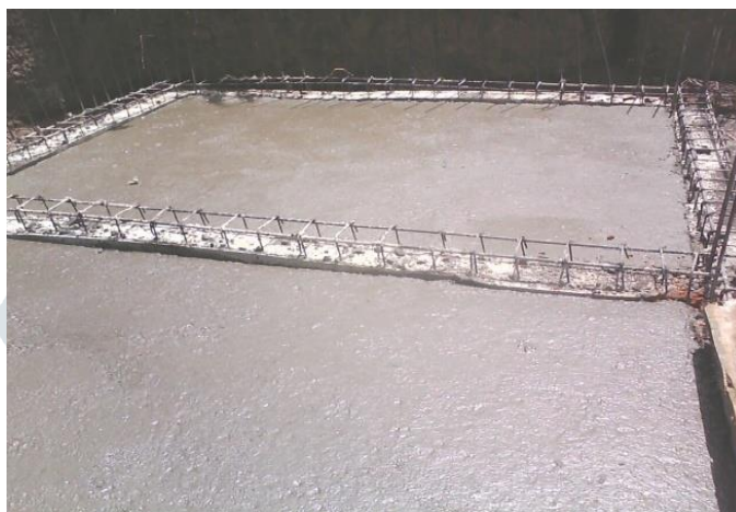
Figure 3: Photograph of Raft slab using fly ash based geopolymer concrete
