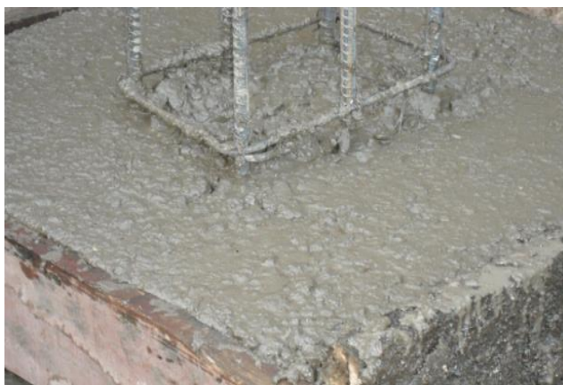
Figure 2: Geopolymer concrete (M30 grade) placed in isolated Footing.
