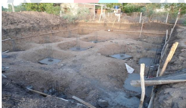
Figure 4: Photograph of different Footings made by geopolymer concrete.
