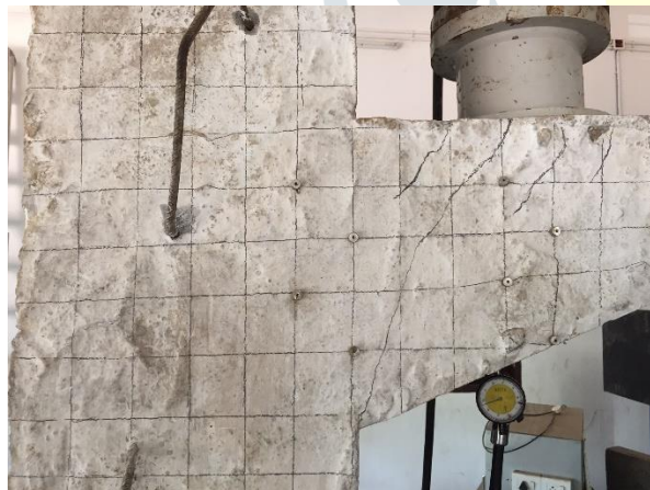
Fig .8: Crack on Specimen with GFRP Bars
