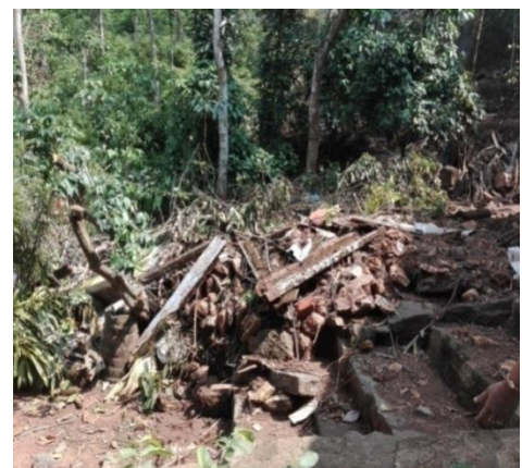
Fig.:1: Slope failure that took place at Kullanpadi- Muttakuzhi, Konni
