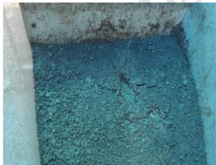
Fig. 11: Failure of slope on stabilizing with 75mm thick geotextile at 133mm/h rainfall intensity
