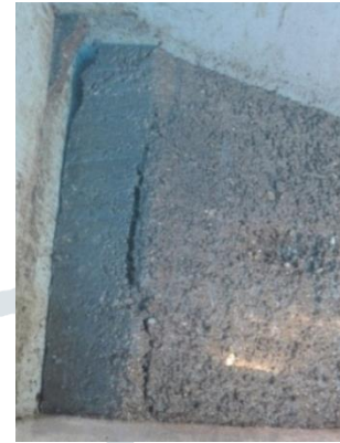
Fig. 8: Failure of slope after 3 hours
