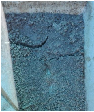
Fig. 10: Failure of slope after 3 hours at 133 mm/h rainfall intensity
