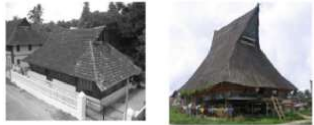
Fig 4. Comparison of Saddle-Hipped Roof of House in Kottayam District, Kerala, India and Batak Karo,
