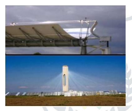
The main principal involved is to focus sunlight on a receiver where the circulating fluid gets heated and there by drives a steam engine to generate electricity.
