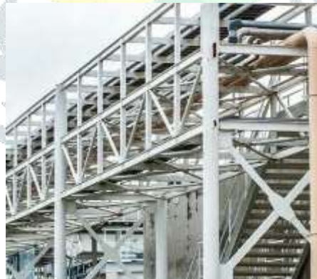
Fig.1 Pipe Rack Structure
