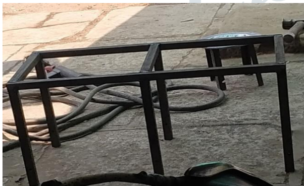
Welding of Square Channel (Base)
