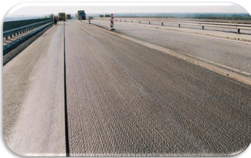
Pavement surface after milling Fig.No.4
