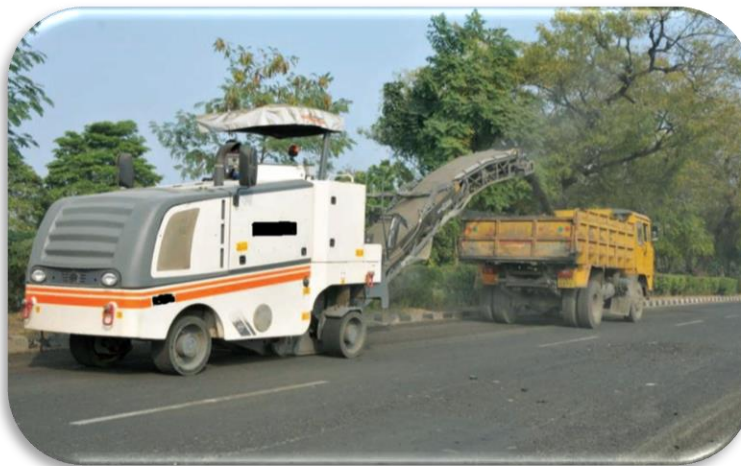
Milling operation at site Fig no.6
