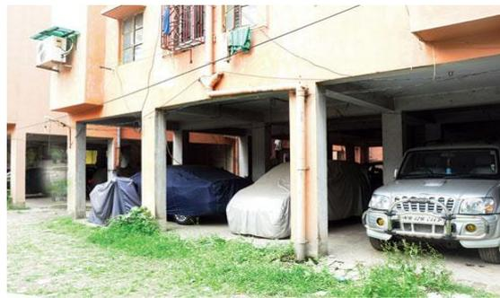
Figure no-1 Open Ground Storey (courtesy –www.telegraphicindia.com)
