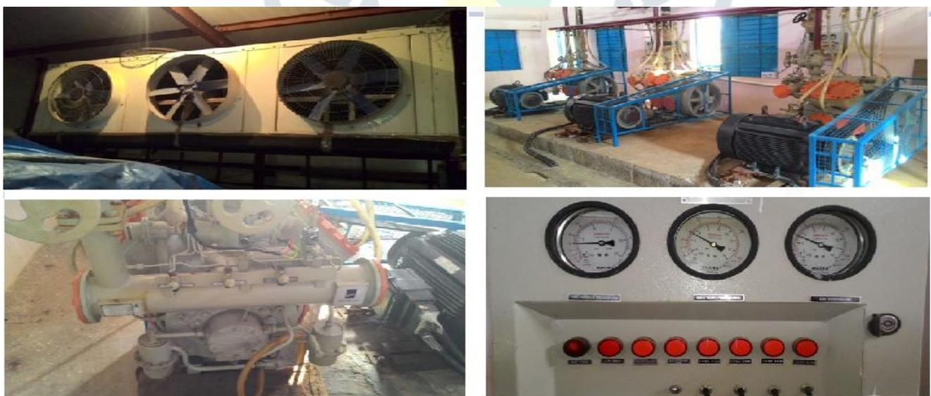
Fig -4: (A) Cooling Fan (B) Compressor (C) Chiller plant (D) Compressor Pressure gauge
