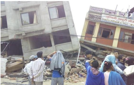
**Fig. 5.** RC Frame structure building collapsed at Sitapaila
