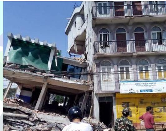
**Fig. 4.** RC Frame structure damage by 12th May, 2015 Earthquake (aftershocks) at Sallaghari
