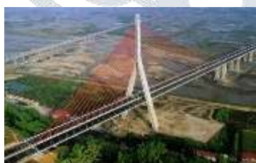
Figure 2. Inverted Y Pylon
