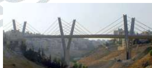
Figure 3. Y-Types Pylon
