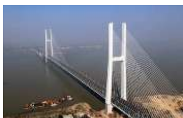
Figure 1. H-Type Pylon
