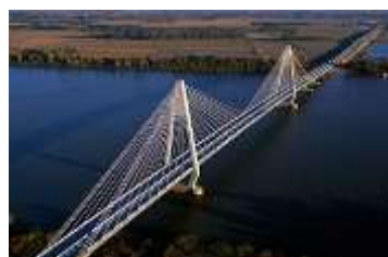
Figure 4. Delta Pylon
