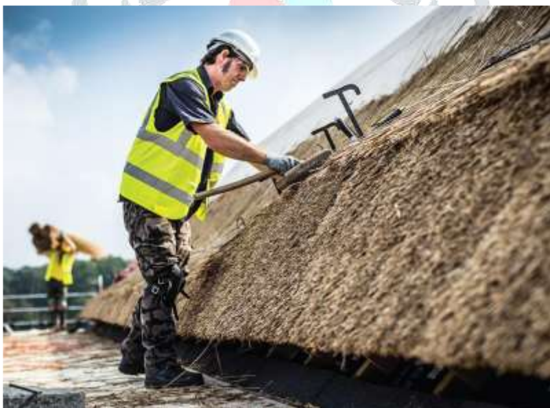
Fig-1: Thatching roof construction
