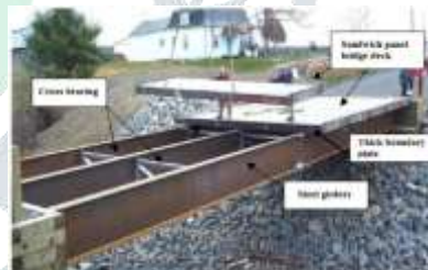
Fig 2 Sandwich panel installation as bridge deck
