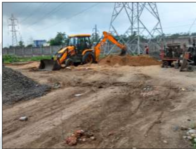
Fig 3.5: Bulldozer bringing sand at work site
