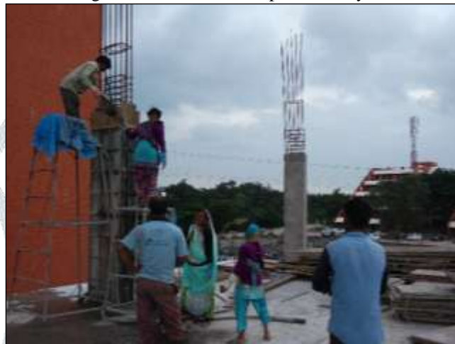
Fig 3.2: Casting of Column
