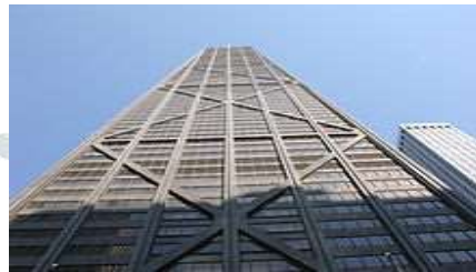
Fig 2.2 Cross Bracing
