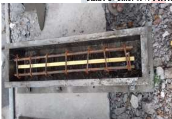
Fig -4: Casting of I-section GFRP beam
