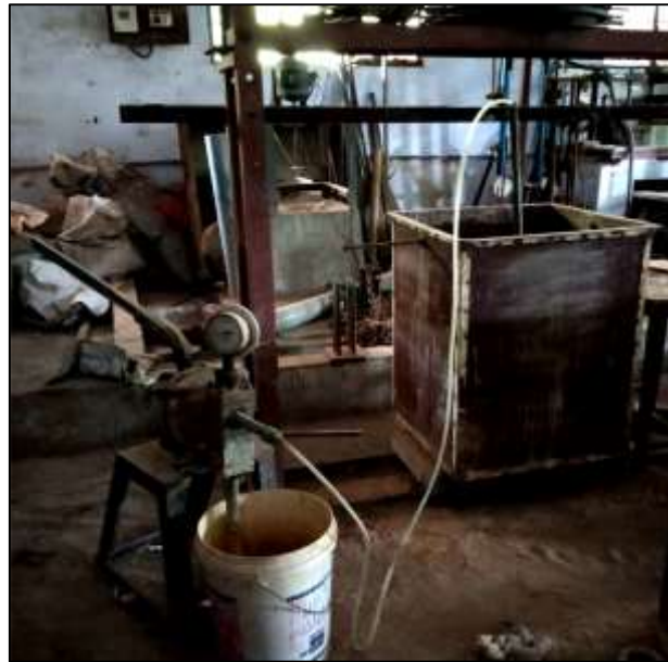
Figure 7: setup for grouting foundation sand mass
