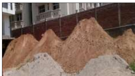
Fig 7- Digging Clay Waste
