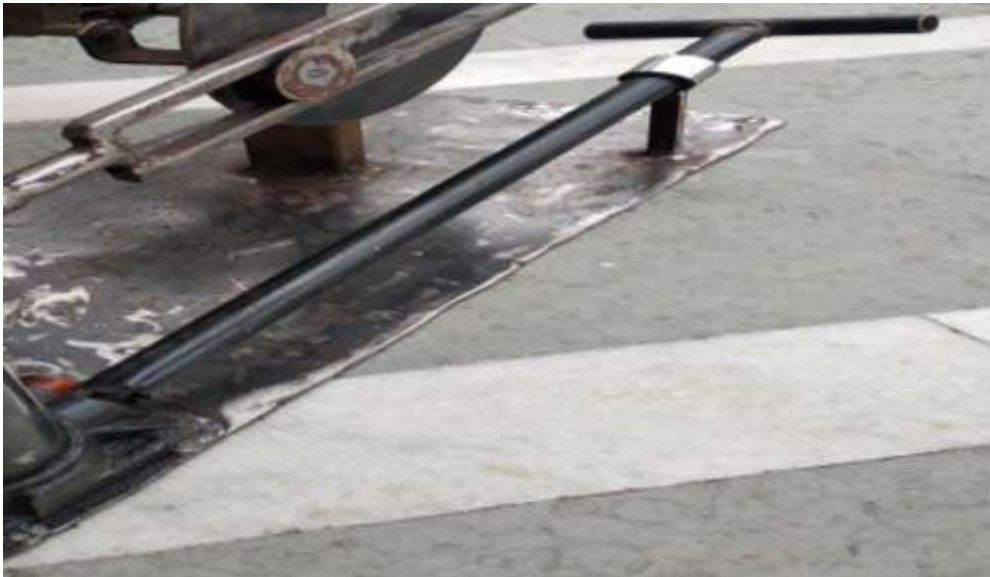
Figure 5 Extension rods for pressure release
