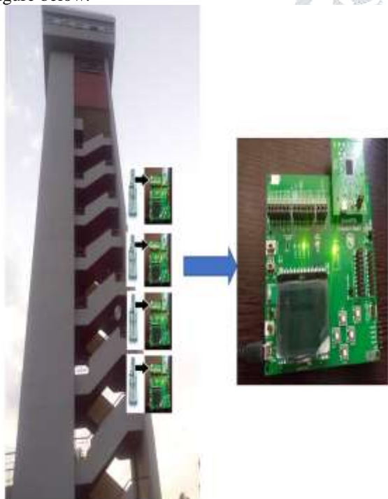
Figure 6.3.1: CEERI TOWER with developed WSN system
