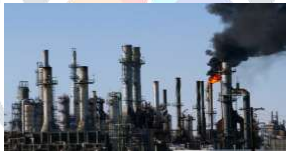
Figure 1.1 Industrial Steel Chimneys (Ref: www.vedomosti.ru)
