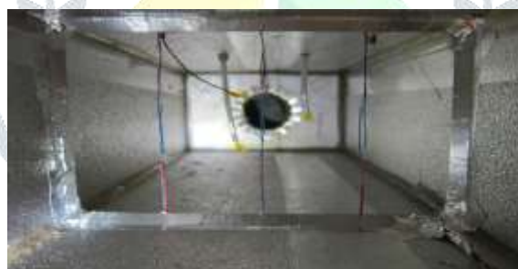
Fig 15: Inside section of channel
