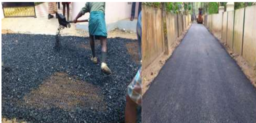
Fig. 5 Laying and compacted finished surface
