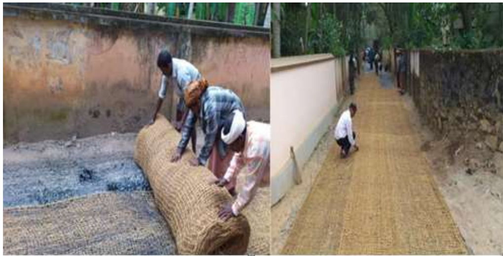
Fig 4 Placing and tying of geotextiles over the prepared surface.
