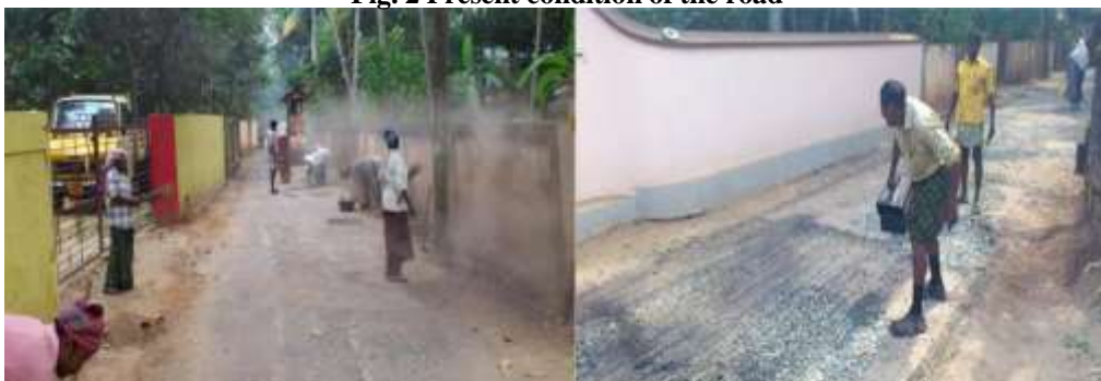
Fig. 3 Cleaning and preparation of the surface
