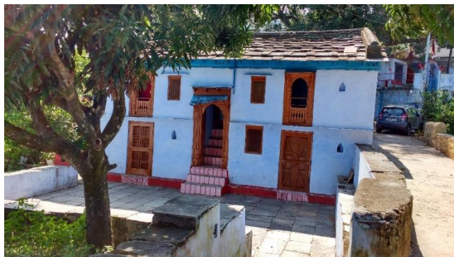
In place of daan (semi open room at ground floor) closed rooms are constructed
