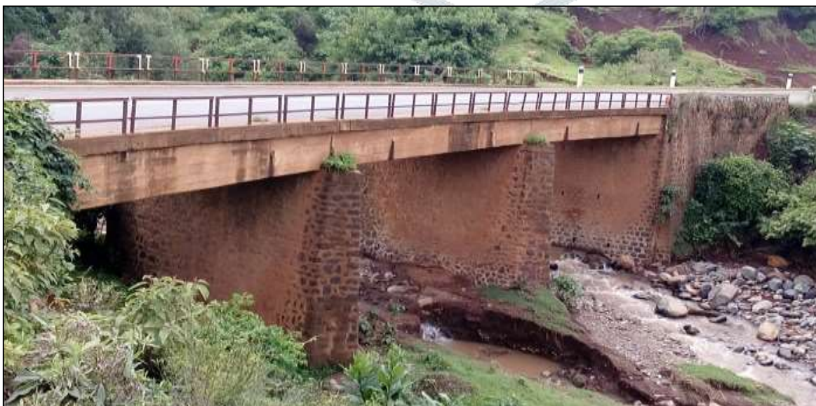
Figure 8. Side View of Oda Bridge
