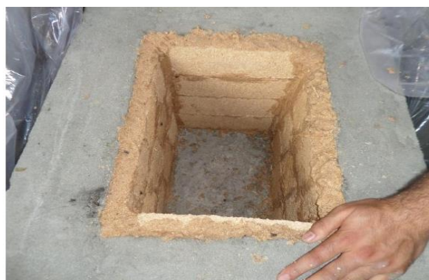
Fig.2. Installation of sawdust tiles in prototype
